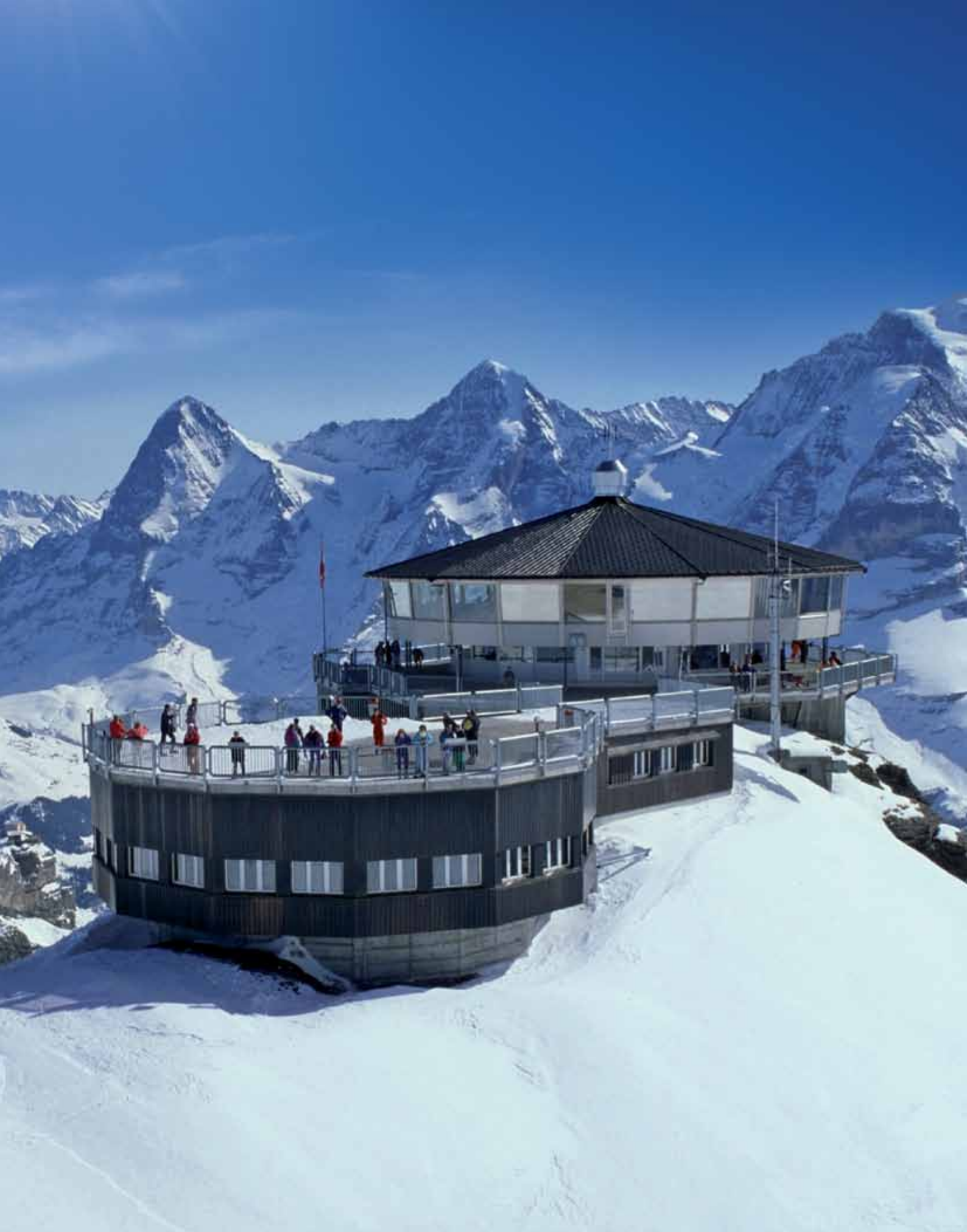
Schilthorn, 2,971 m above sea level, Switzerland, PREFA anthracite roof tiles.
